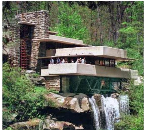
Figure 47 Fallingwater View to NW - Note Steel Braces Under Balcony
