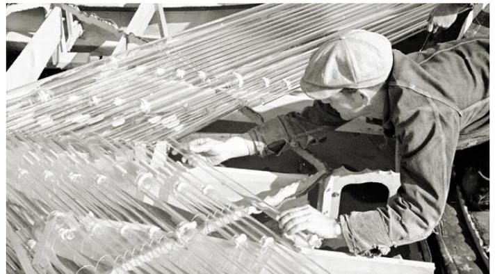
Figure 13 Installing Pyrex Tubing in the Skylights of Headquarters c.1938
