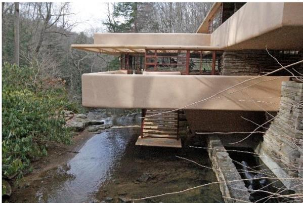
Figure 48 Fallingwater View Downstream prior to Steel Bracing
