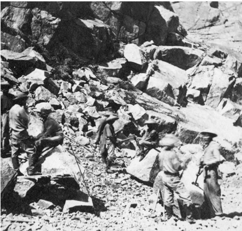
[Originally a stereocard] Plate number 119 by Alfred A. Hart in California circa April 1868. Laborers use tools to chip at the rocks near the opening of the Summit Tunnel. Part of the "Scenes in the Sierra Nevada Mountains" stereocard album collection.
