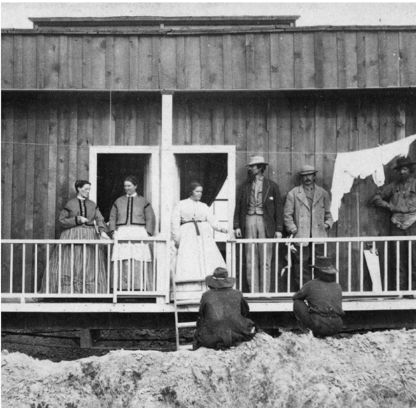
[Original format is a stereocard] Plate number 325 by Alfred A. Hart in Nevada circa November 1868. James H. Strobridge, superintendent of construction, family boxcar. Part of the "Scenes on the Humboldt River" stereocard album collection.
