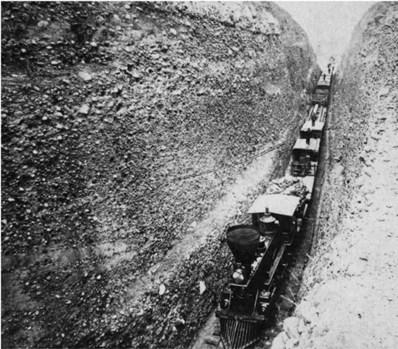
[Original format is a stereocard] Plate number 231 by Alfred A. Hart in California circa June 1865. A train, with men standing on the cars, moves through Bloomer Cut near Auburn, California. The cut is 800 feet long and 63 feet high. Part of the "Scenes in the Sierra Nevada Mountains" stereocard album collection.
