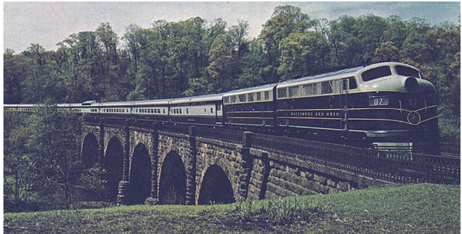
The Columbian on Thomas Viaduct, Relay, Maryland, in 1949
