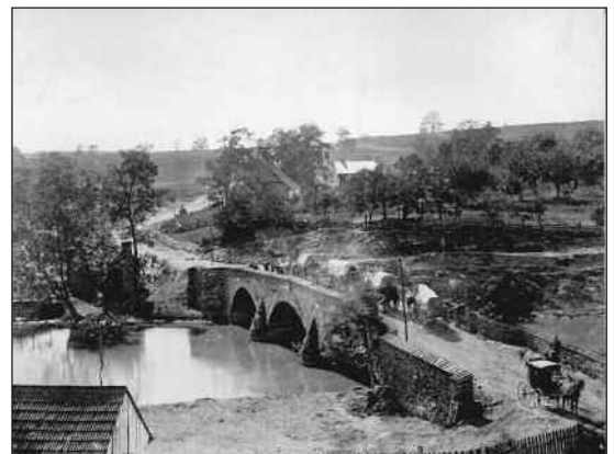
Soldiers and wagons crossing the Antietam Bridge, 1862
